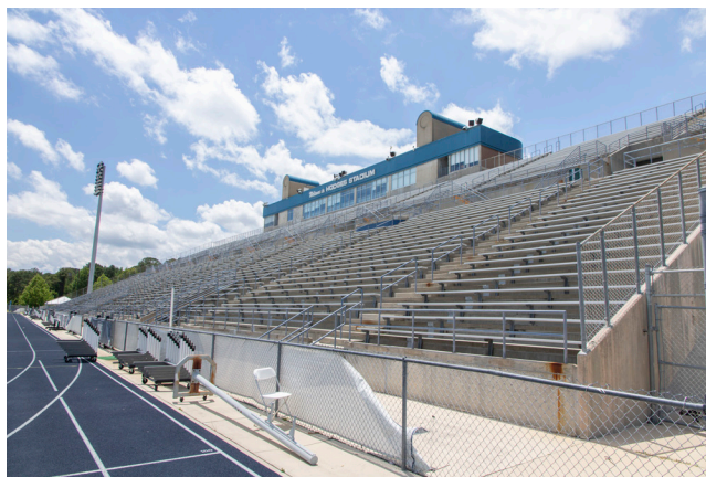
Harmon Stadium is the largest outdoor athletic facility on campus and was constructed in 2000
