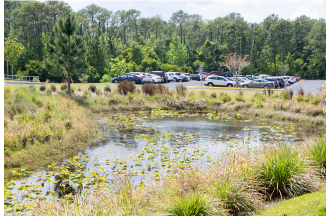
UNF has a number of stormwater ponds across the entire campus, supplemental to existing stormwater infrastructure.
