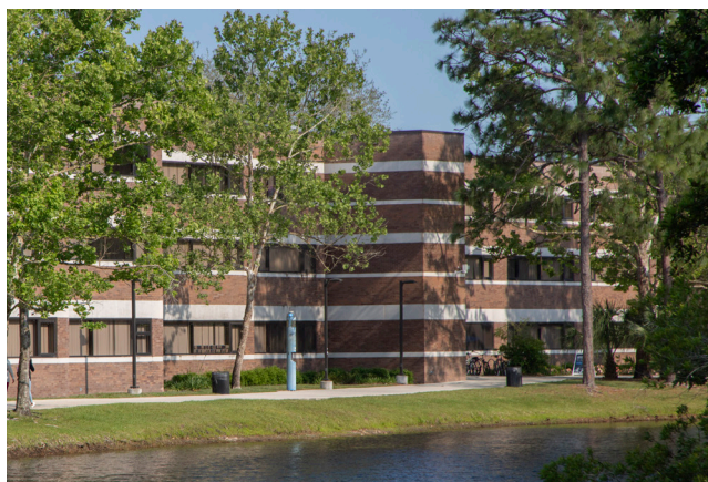
A number of older buildings on campus have maintenance issues or would be difficult to renovate to meet modern needs
